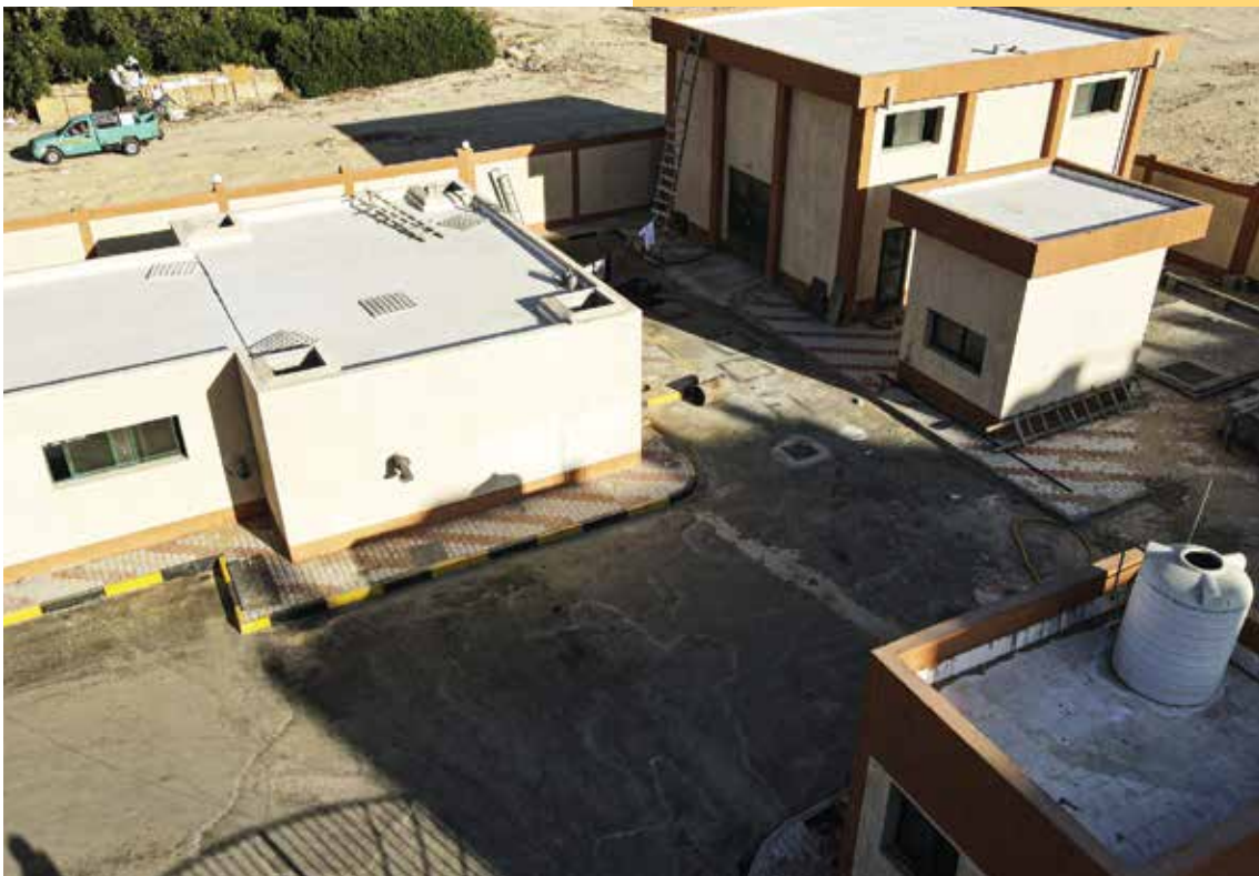
Irrigation water pump station-Hurghada Holding Co. For Water & Wastewater (HCWW)
